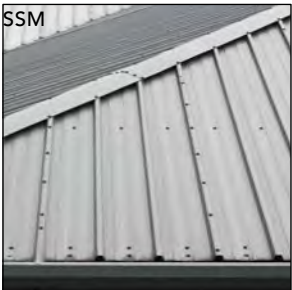
Metal Roofing Type: Standing Seam
