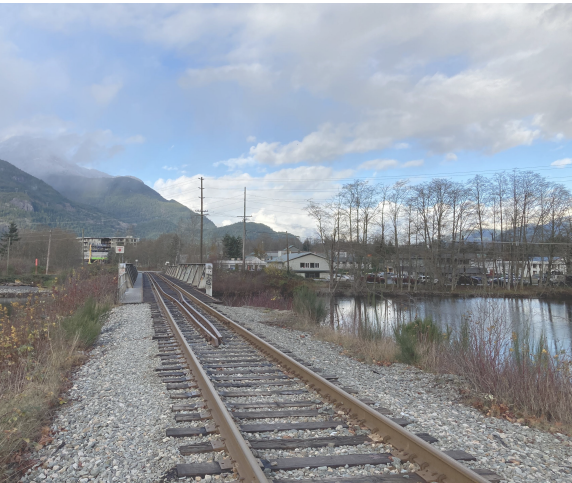
Mamquam Blind Railbridge Looking North Towards Development
