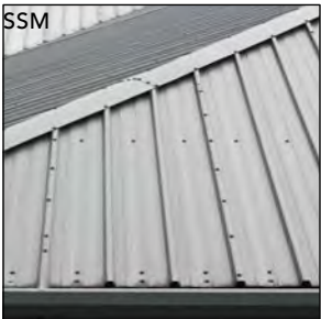
Metal Roofing Type: Standing Seam
