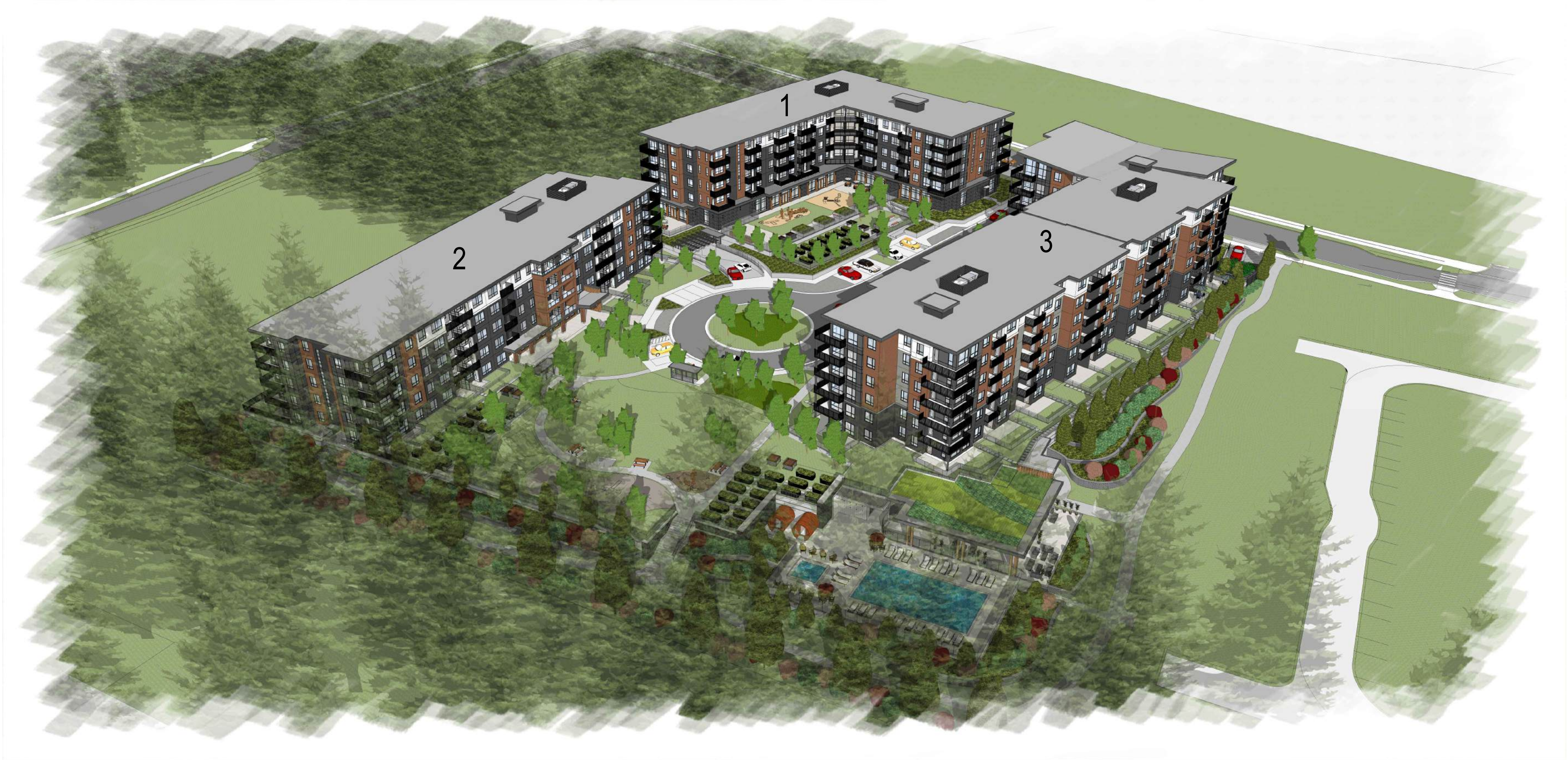
AERIAL VIEW - LOOKING NORTHEAST
