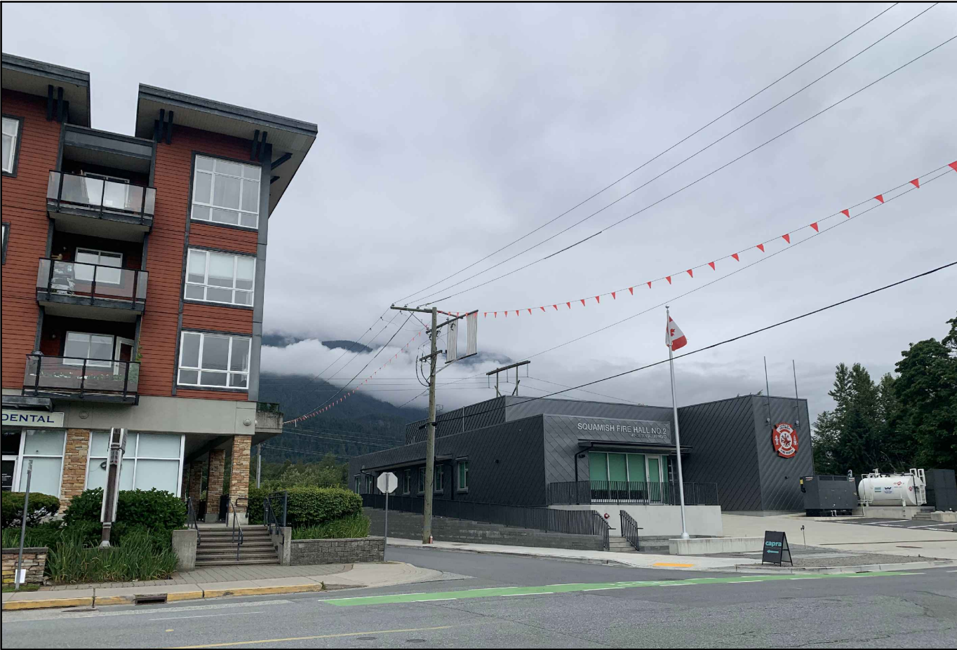
1 FIREHALL, SOUTH OF SITE
