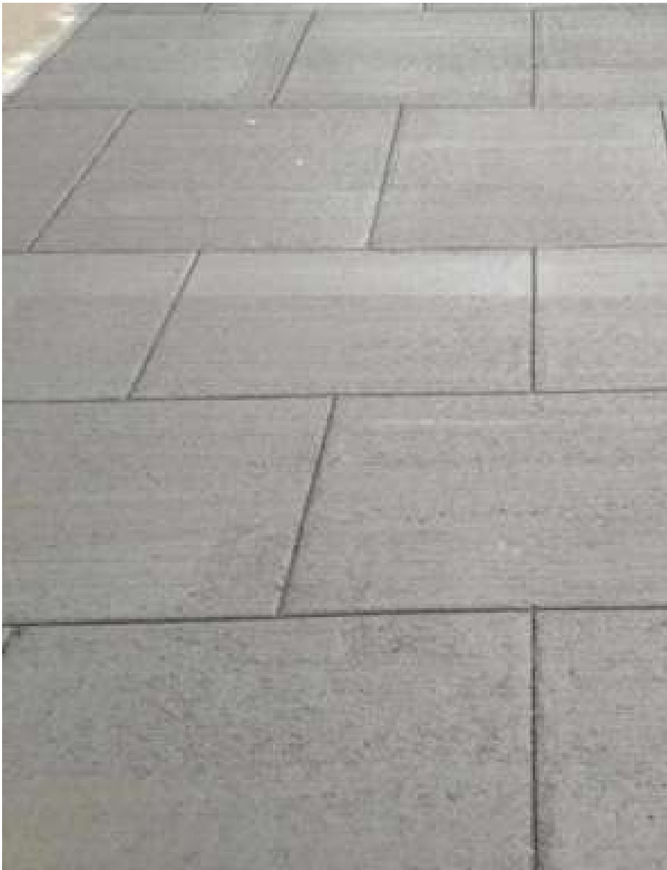
CONCRETE PAVING W/ SCORING PATTERN
